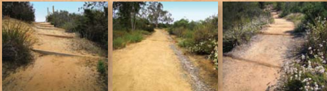
Water Bars Gravel Trenches Rain Channels
